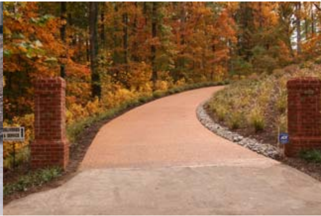
Drive Entrance After
